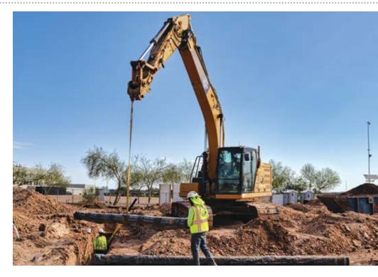
"On one project in particular, there were four plan revisions after we started, and you can't update the model fast enough to keep up with those changes," Campbell says. "So that's where the laser catcher and the grade controls come in and help resolve the missing links. The system is integrated in the machine, and enables us to make those adjustments in the field and still maintain accuracy and productivity."
